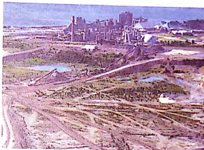
A cement plant – the site was chosen because of the availability of limestone shale, coal and water.
